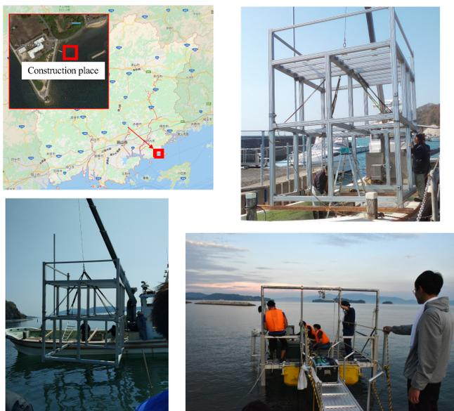
Fig. 2 Permanent stage for underwater robot experiments and installation procedure and the location
